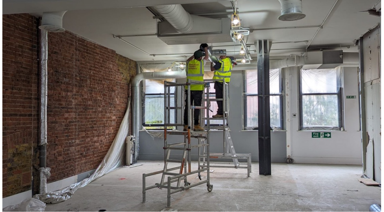
↑ Ductwork simplified throughout to reduce visual noise
