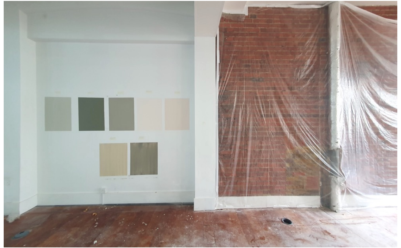
↑ Paint work samples for both standard smooth finish and artisan limewash finish. Earthy, neutral palette throughout.
