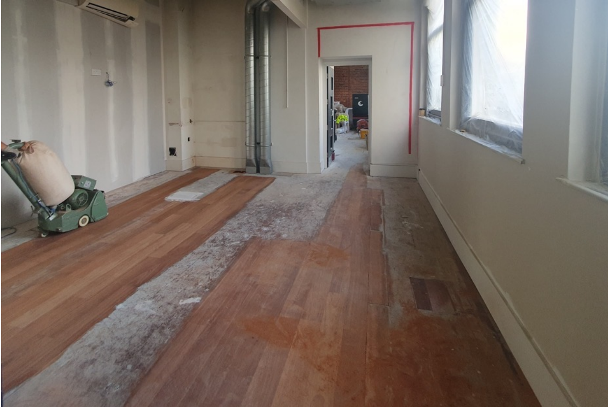
↑ Restoring the original Merbau hardwood boards throughout the Ground Level
