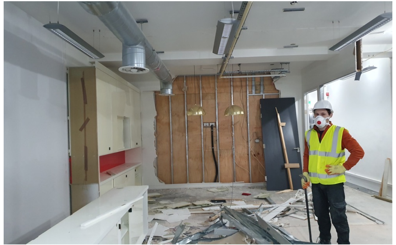
↑ Courtyard Level: early soft strip stage
