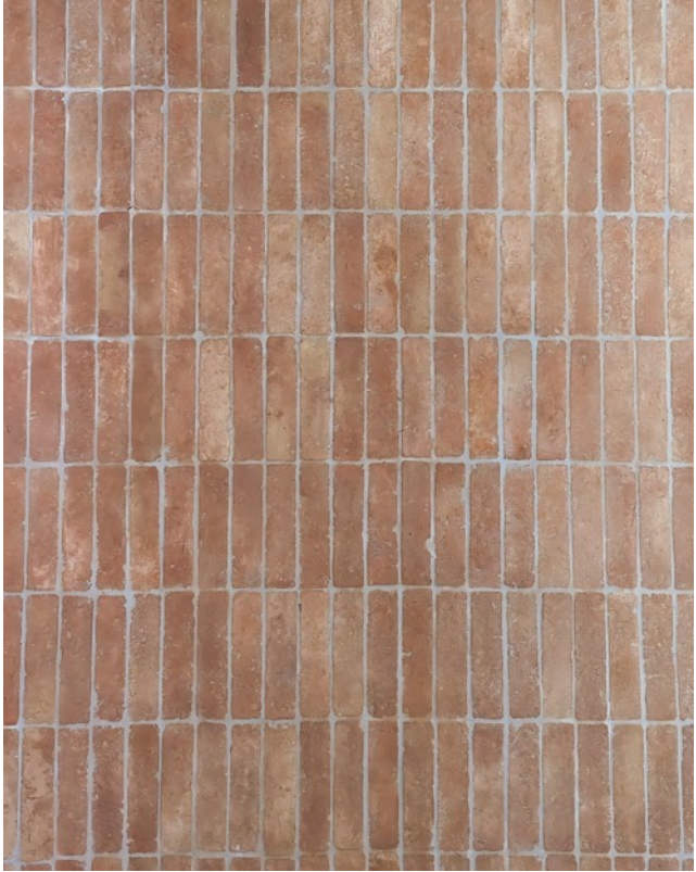
↑ Courtyard Level: 18,480 hand-installed terracotta tiles, sourced from Artisans of Devizes – to last another century
